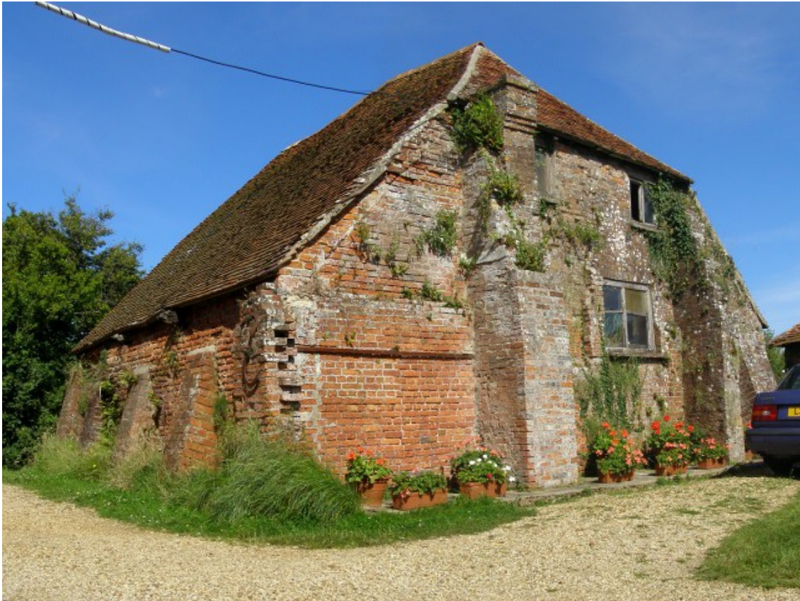
Listed Salt Barns adjacent to Creek Cottage, Moses Dock Pennington
